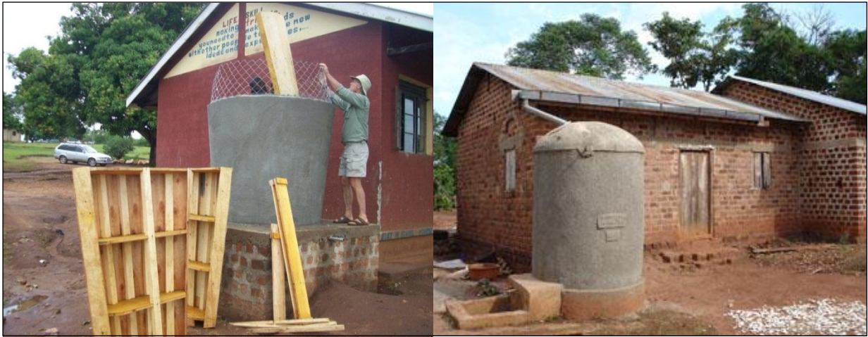
Figure 1.10: First rain water harvesting concrete tank source: installation
