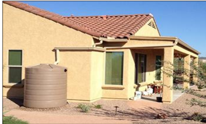
Figure 1.9: Plastic Rainwater Harvesting Tanks source Southern Arizona Rain Gutters Southern (source: Arizona Rain Gutters)
