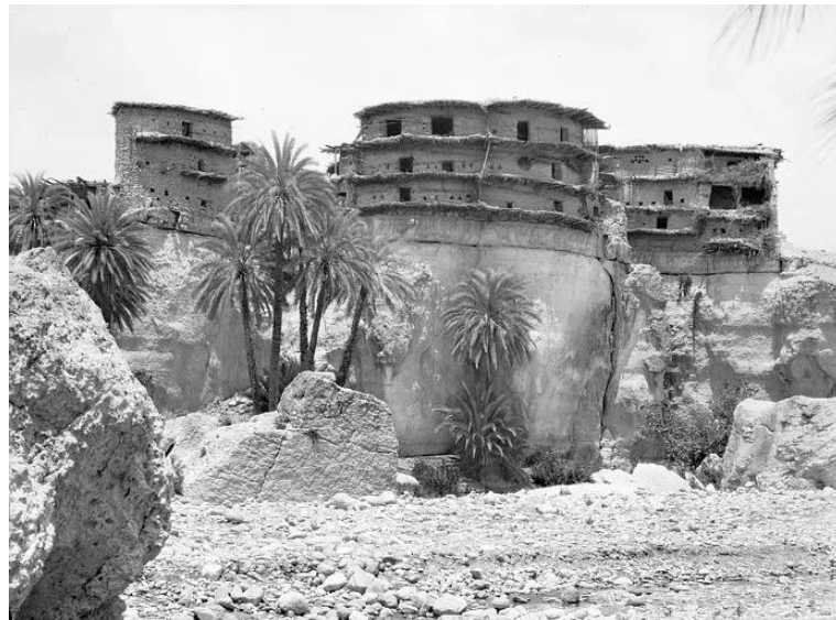
Figure 9 : Grenier fortifié de Houkhribth - Ibanyene - Aurès Source: Copyright (C) www.facebook.com/Inumiden
