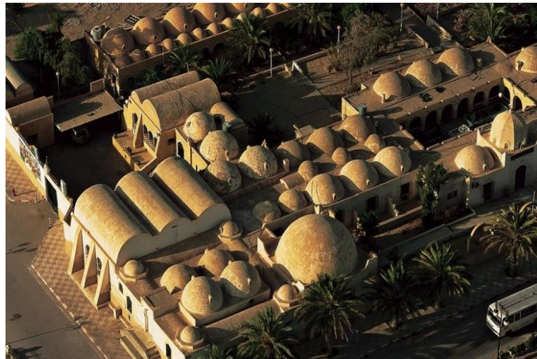
Figure 1. Domes and vaults used in El-Oued (capital of the Souf region)
