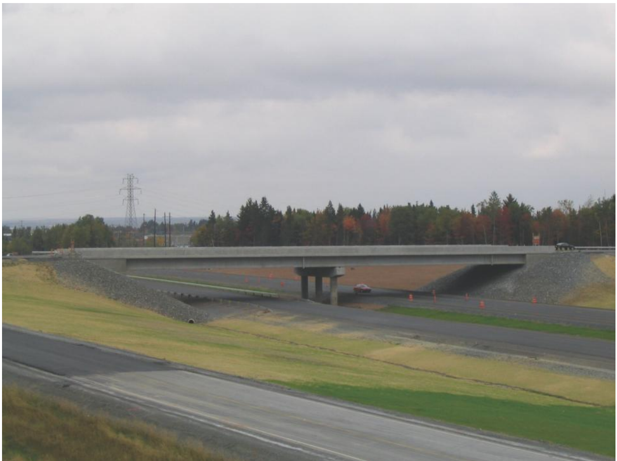
Figure 1. 10. Full scale monitoring bridge - "Route 2 high-speed connector underpass" New Brunswick – Canada
