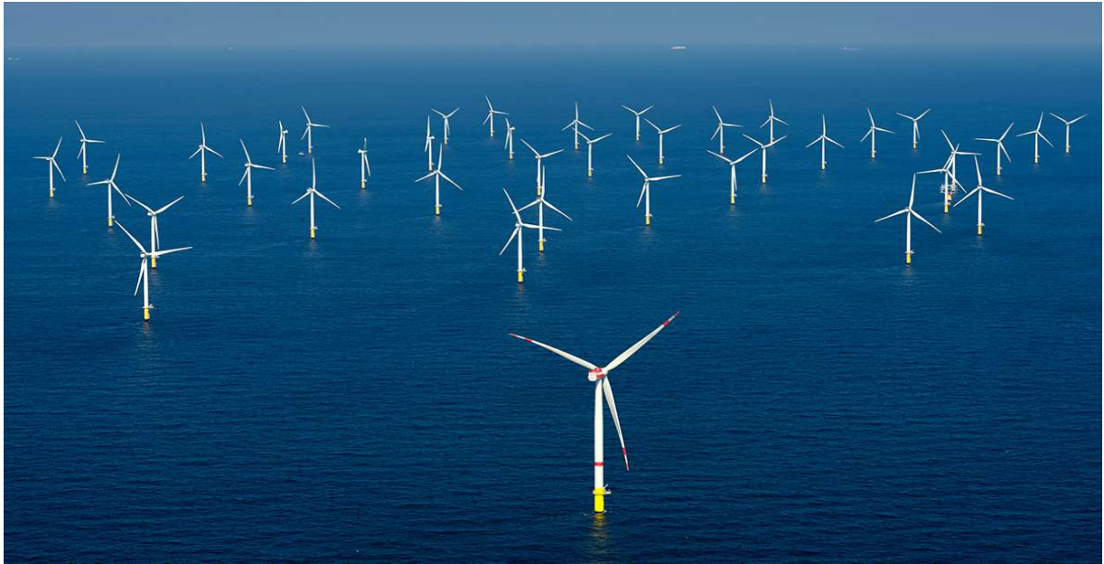
Figure I.6 Offshore wind turbines [46].
