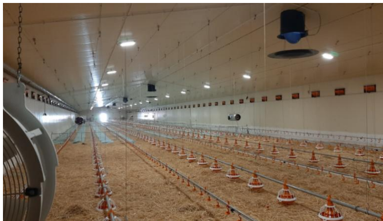
Figure 2.4. Actual photo inside the building shows part of the systems used in it.
